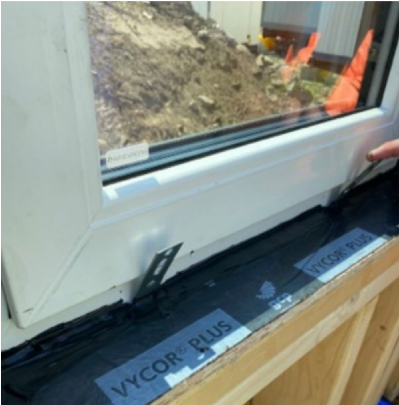
Interior Seal top and bottom at clip
