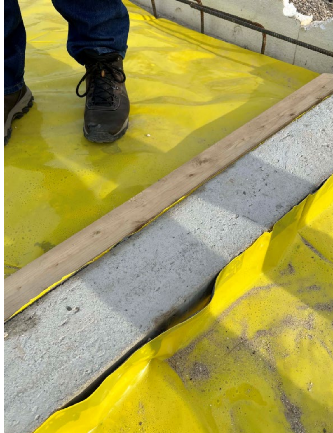
There are different products for sealing the vapor barrier. Conduit and plumbing penetrations require coordination.
