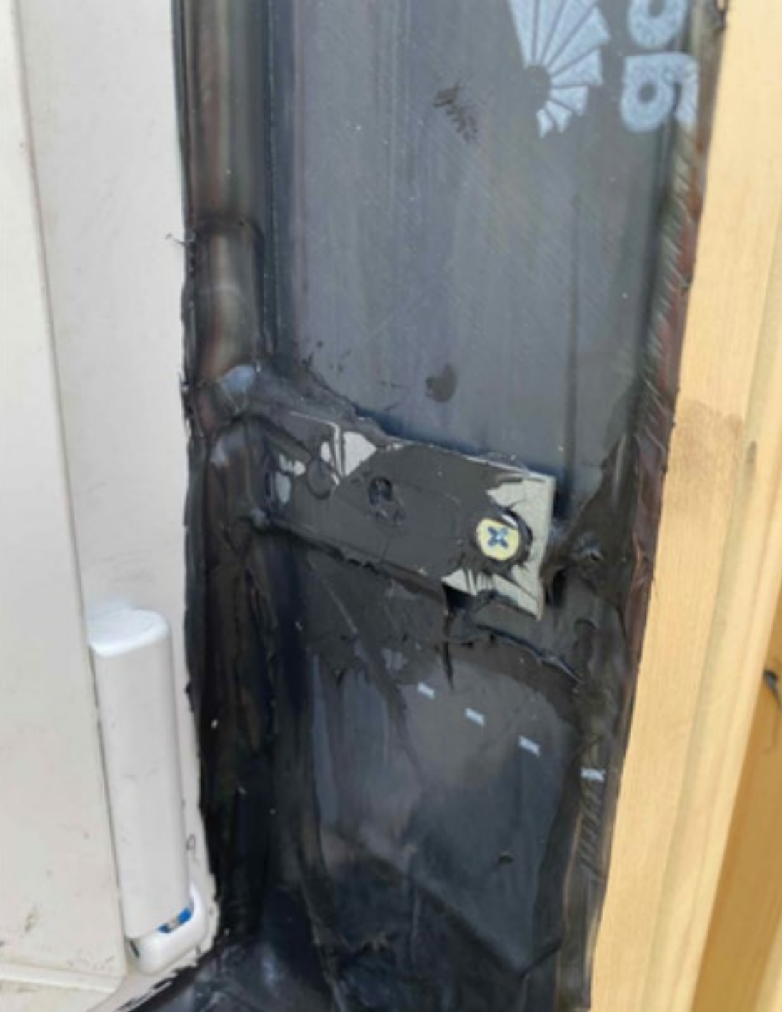
Interior Seal at Clip – Set in sealant
