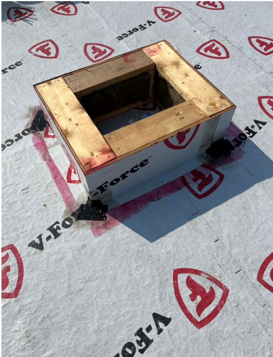
Good air seal, but the insulation or lack thereof, needs work.
