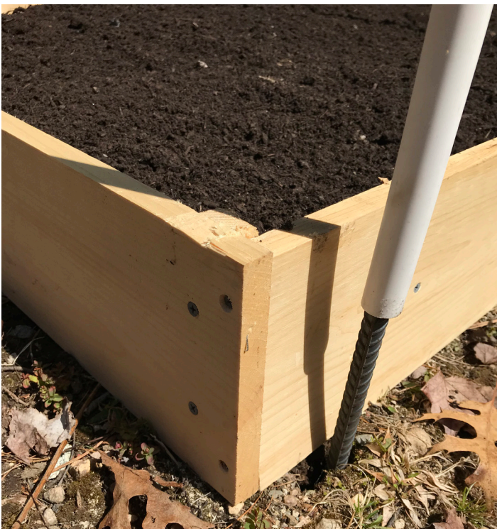
Figure 5 Rebar anchors for PVC pipe
